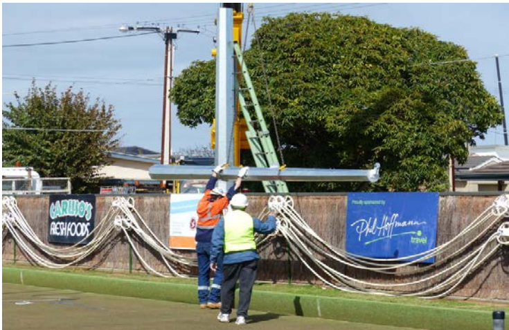
Working on the light poles.
