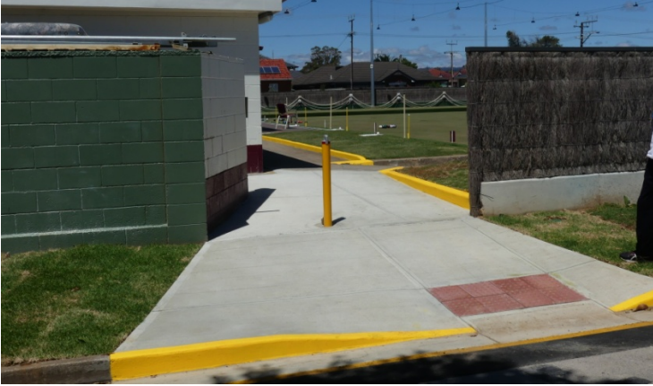
The disabled walkway on the western boundary.
