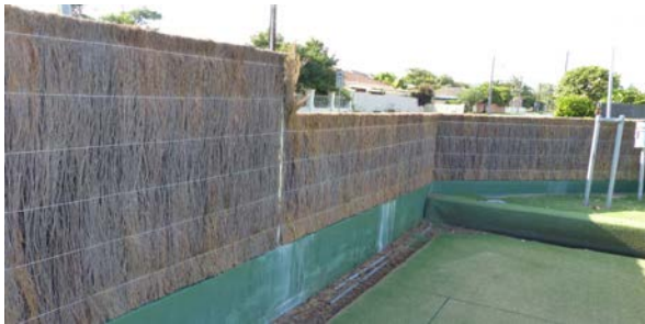
The newly constructed southern perimeter fence.
