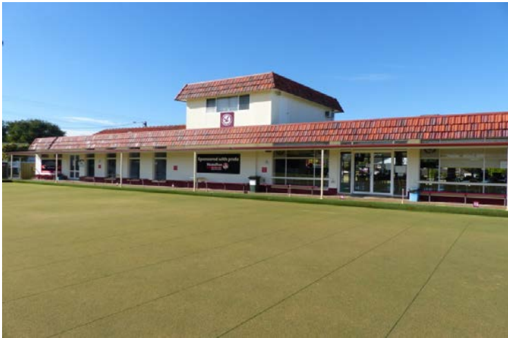
A newly renovated clubhouse.
