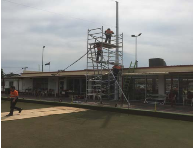
Plywood sheets used to prevent damage to the greens.
