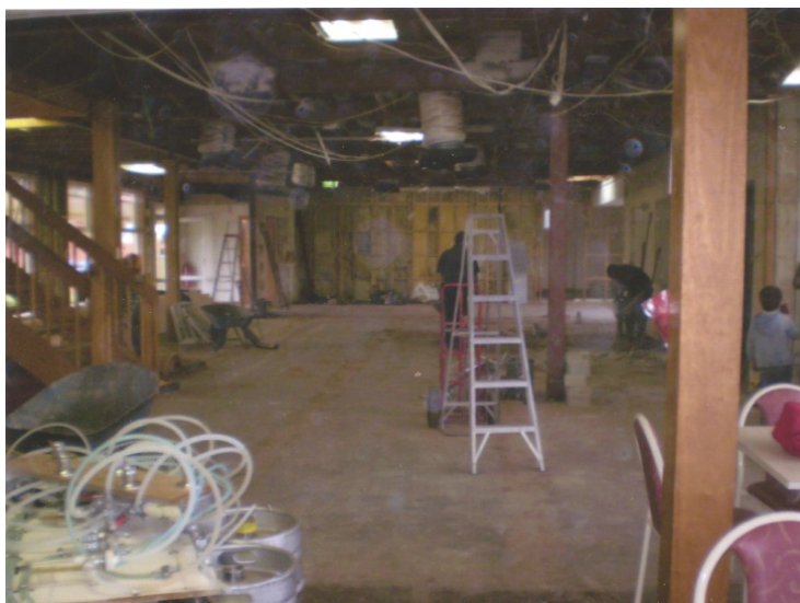
Demolition of the old premises before renovation.
