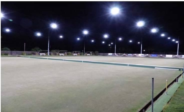
New lights installed over A and B greens.
