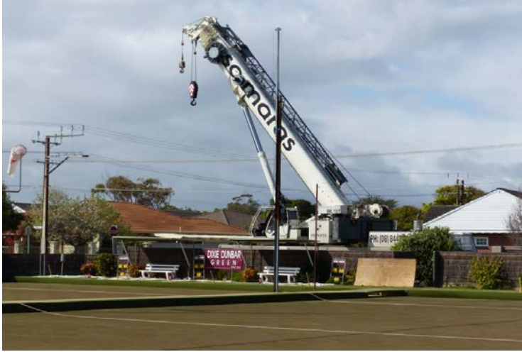
Heavy equipment used to hoist light poles into position.
